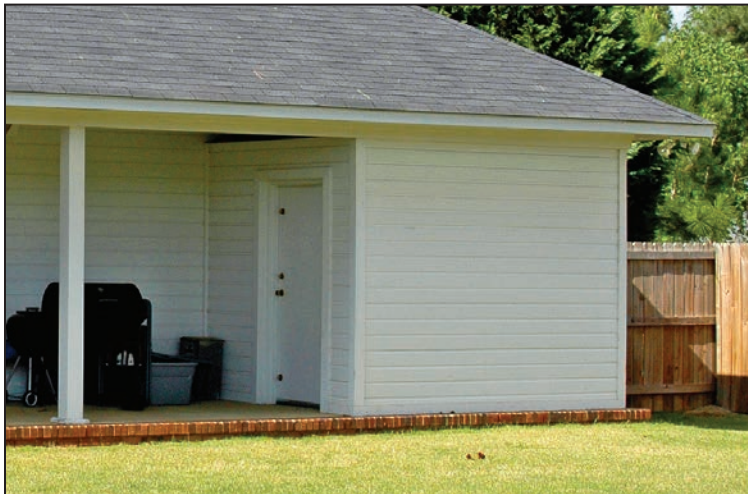
Figure 3-5: An above-ground safe room constructed as an addition to a slab-on-ground home in a way that matches the aesthetics of the house (outside Tuscaloosa, AL, 2011)
